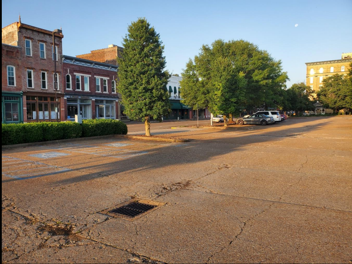
South portion of site, facing SW
