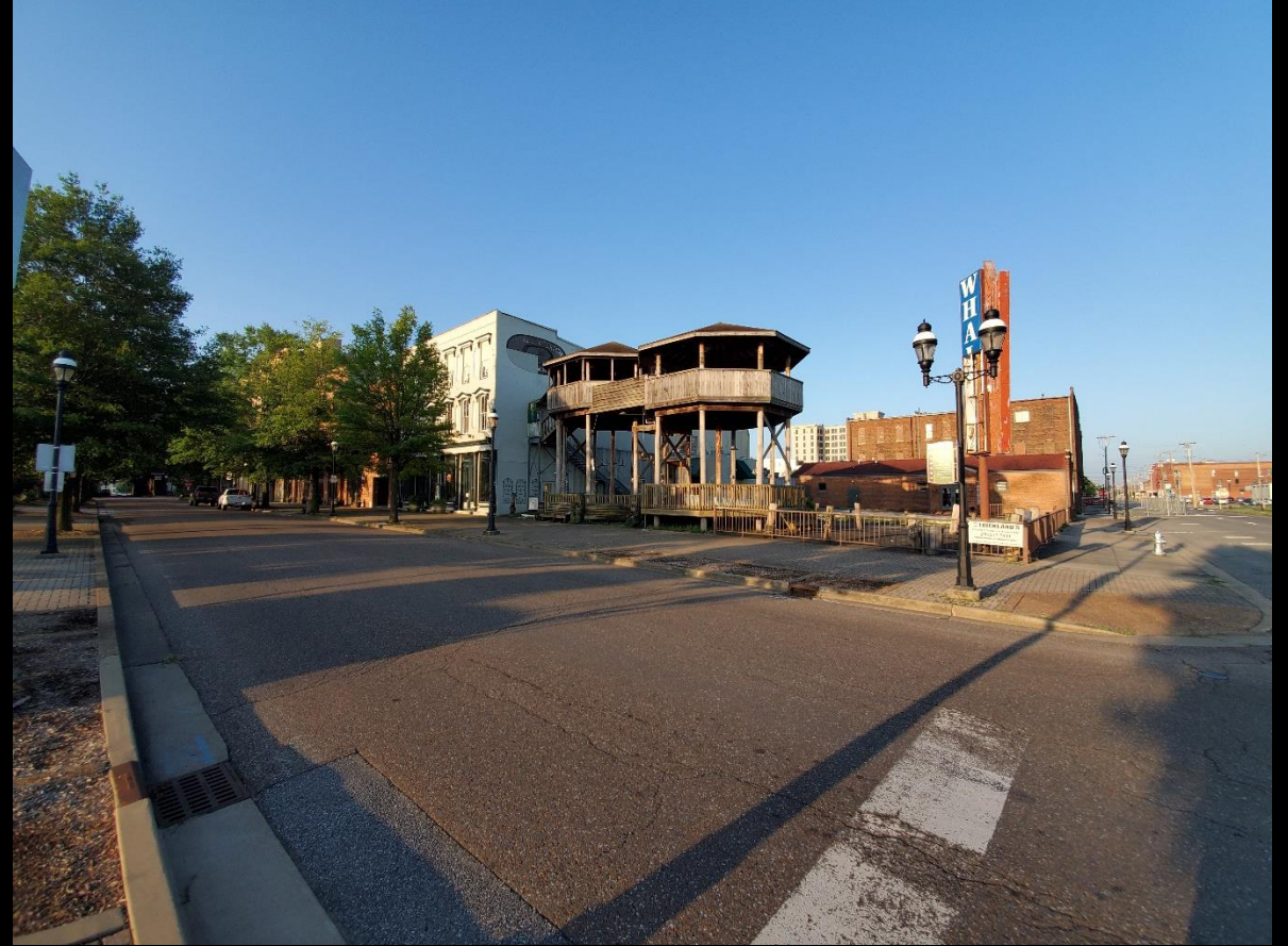
NW adjacent property, facing SW
