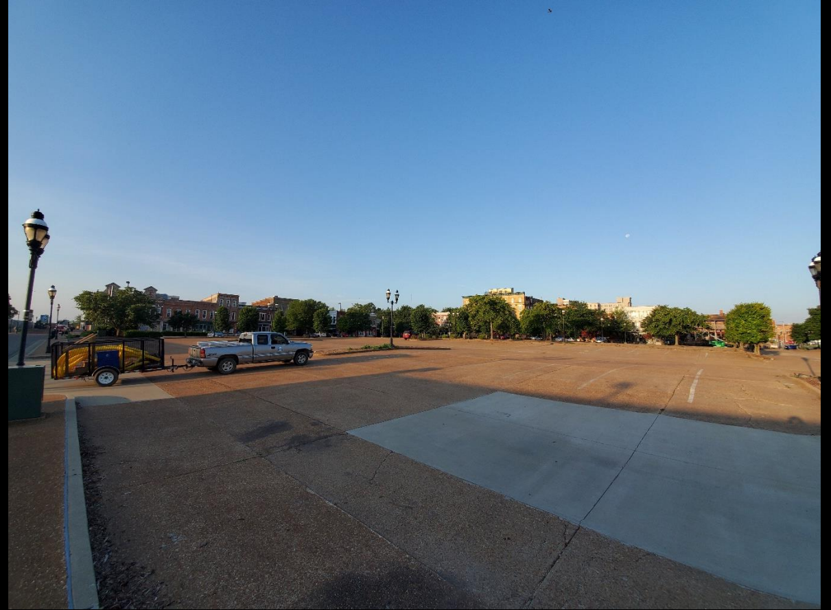
NE corner of site, facing SW
